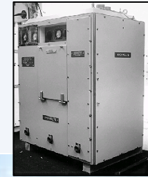
Rod control gear & pressuriser heater controller
