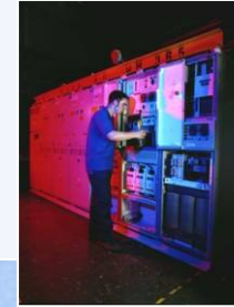
Rod control gear & pressuriser heater controller
